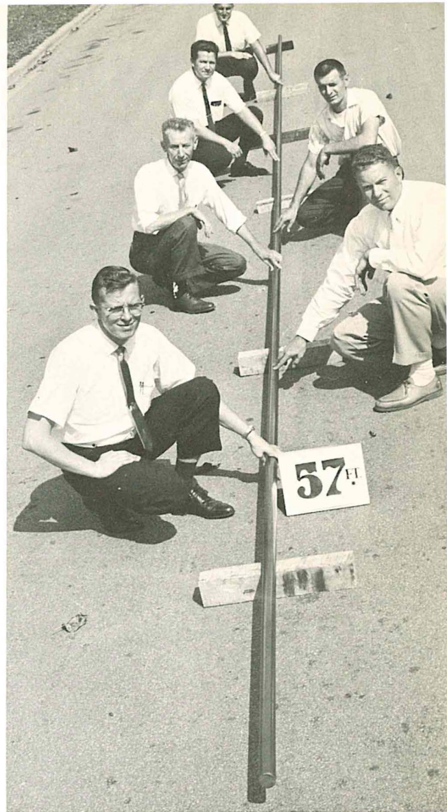
Fifty-seven feet of cold steel, longest bar ever drawn in the industry, is displayed by company officials at Nelson Steel & Wire Co., Franklin Park, Illinois. The record bar is 2" in diameter and weighs 610 pounds. Before cold drawing the bar was descaled in a three-wheel Wheelabrator Cabinet which provides a cleaner finish and brighter bar than can be obtained by pickling.
